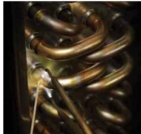
Brazing of copper return bends
